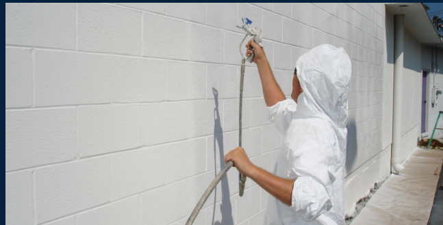
Applying ThermaCote® to the exterior wall of cmu block on this dance studio in Atlanta, Georgia stopped 'breezy' air infiltration and wide temperature swings inside while also being aesthetically pleasing.
