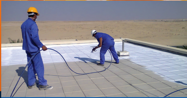
ThermaCote® being installed on a 'concrete tile' deck of a roof in Dubai
