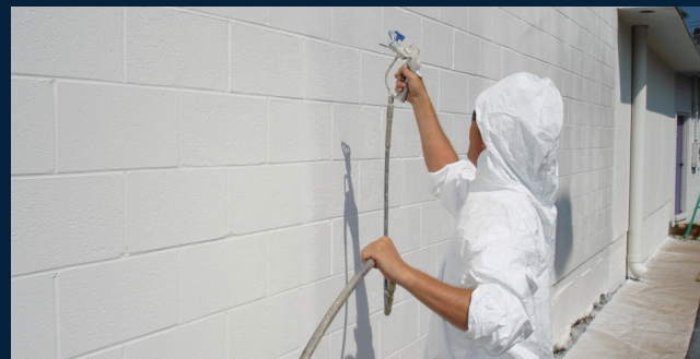
Applying ThermaCote® to the exterior wall of cinder block on this dance studio in Atlanta, Georgia stopped 'breezy' air infiltration and wide temperature swings inside while also being aesthetically pleasing.
