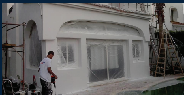
ThermaCote® during installation on a villa in Casablanca, Morocco
