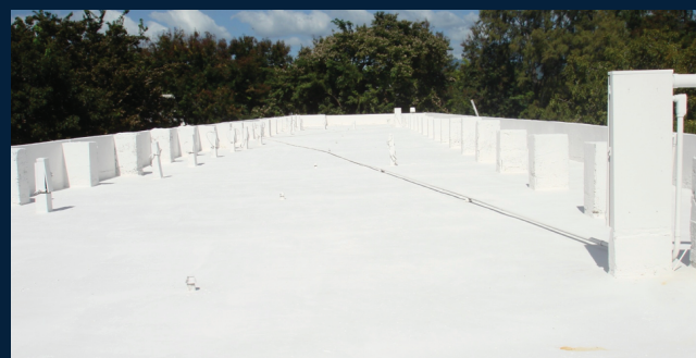
ThermaCote® applied directly to a concrete roof of a university in Puerto Rico
