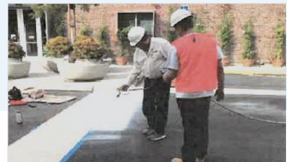
ThermaCote® installation on asphalt for the Los Angeles Cleantech Incubator test
