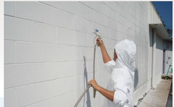
Applying ThermaCote® to the exterior wall of a CMU block at an Atlanta dance studio. This stopped air infiltration and wide temperature swings while also being aesthetically pleasing.
