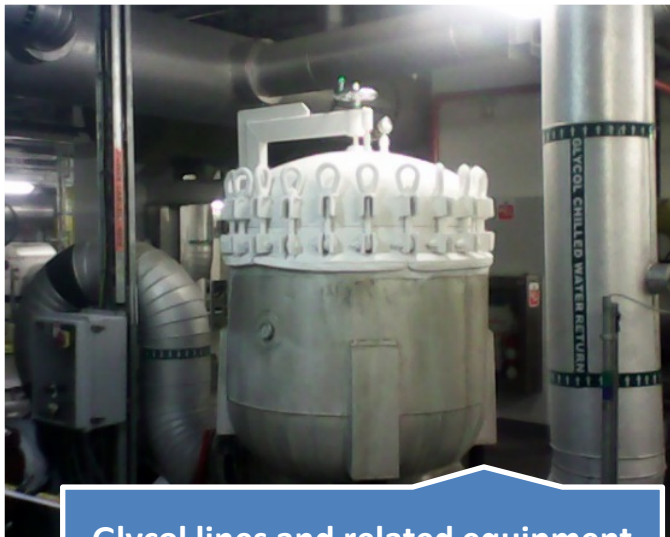
Glycol lines and related equipment for the cooling system with ThermaCote for Dubai Airport
