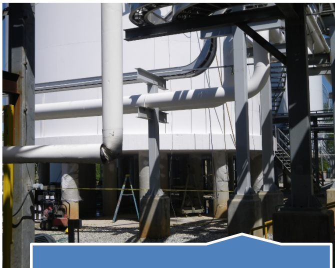
Liquid oxygen Pipe Insulation
